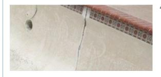
"When we see a structurally cracked pool, it's usually pretty obvious. It's a crack running either down the side of a pool from the tile or through the bottom coping down the walls, across the floor, in corners, and very often, it's opened up enough that it can leak and bring water in. It'll suck a lot of water through that crack because it is broken all the way through, and the water just goes back to the dirt on the back side of the shell."
